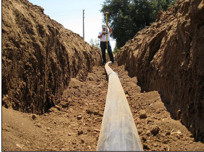
Figure 6.2 Coordinating the pipeline (Web 4)
